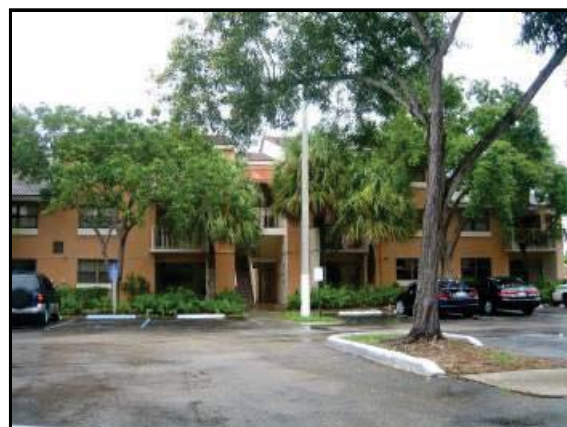
Location: CompListing1 Description: FRONT
